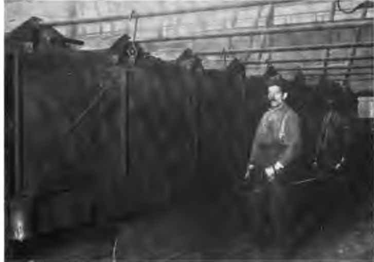
Fig. 2. Screens in Front of Rod Mill Reels.*
